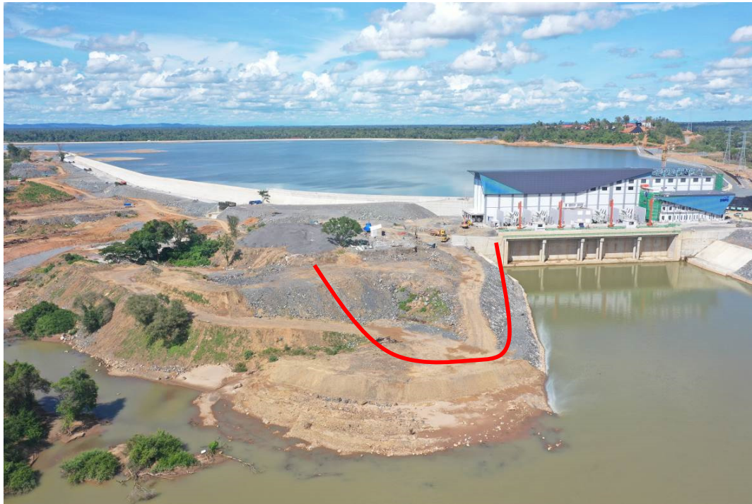
Figure 11.3-1 The axis position of cofferdam
