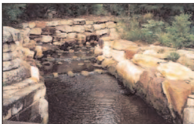
A nature-like fishway built to allow fish to pass a small weir in Australia, successful mitigation in practice
