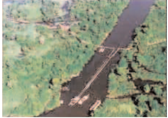
A barrage in flooded forest, built to catch migrating fish
