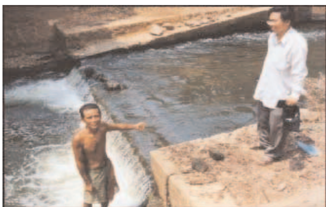
A small drop-structure, a barrier which with better design could allow migrating fish to pass
