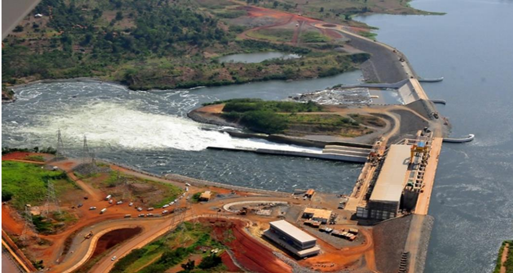
Figure 6.2. General view of the Bujagali Hydropower Project, Uganda (Source: Multiconsult).
