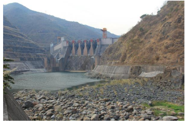
Figure 2.4. Dachaoshan Hydropower Project (Source www.flickr.com ).
