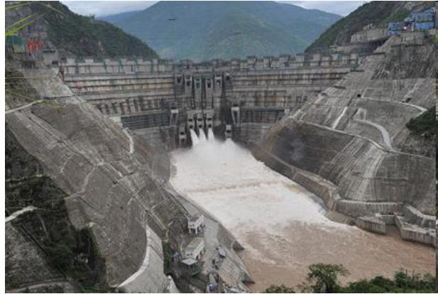
Figure 2.6. Xiaowan Hydropower Project. (Source: Mekong River Commission).
