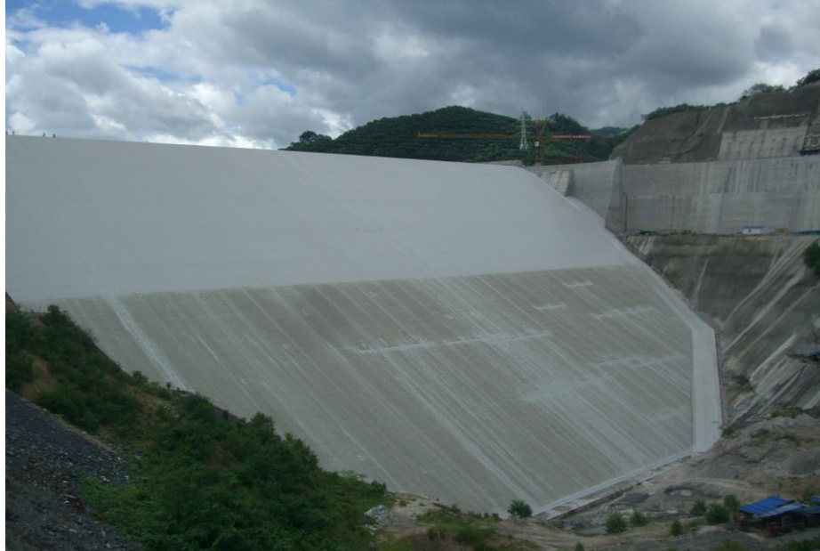
Figure 6.1. Upstream face of the Nam Ou 6 dam, Lao PDR (Source: Multiconsult).
