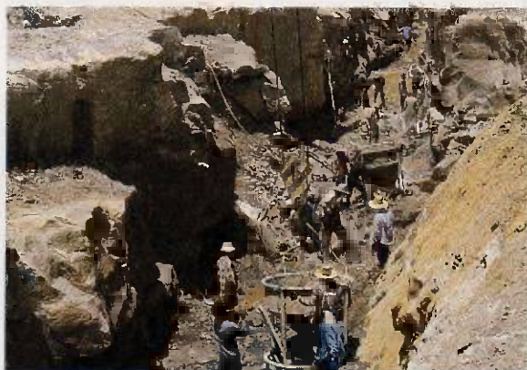
◆ Excavation of diversion channel Huai Pa Thao
