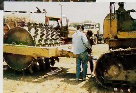
◆ Dike construction at Sithantai
