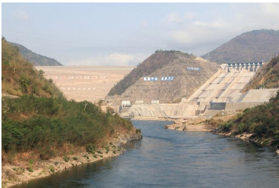
Photo 2-2 Nuozhadu Hydropower Project (Source www.flickr.com )
