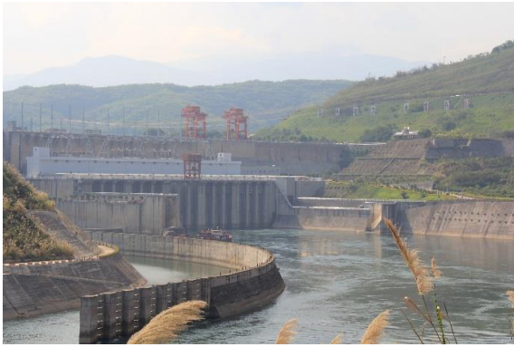
Photo 2-1 Jinghong Dam (Source www.flickr.com )
