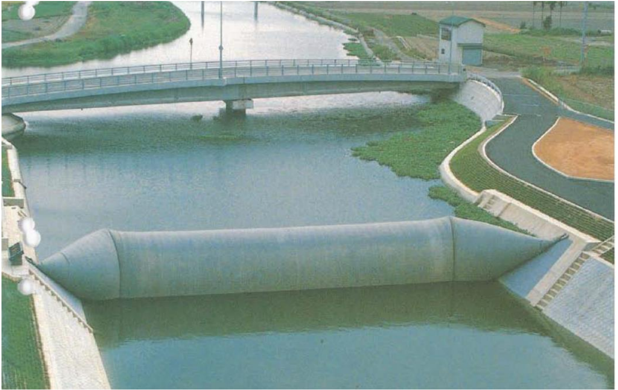
Figure 15: Air-filled Rubber Gate
