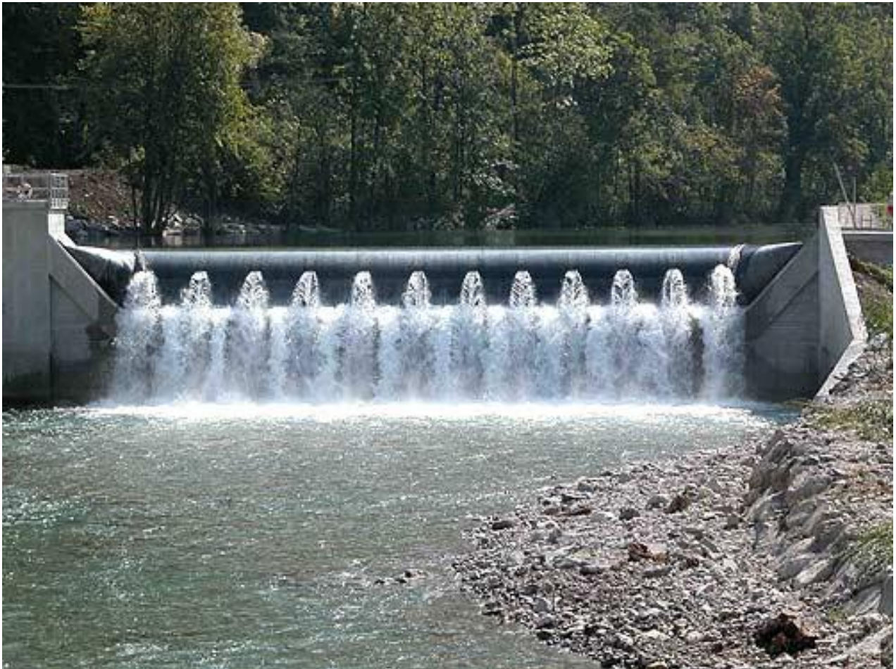
Figure 14: Water Filled Rubber Gate
