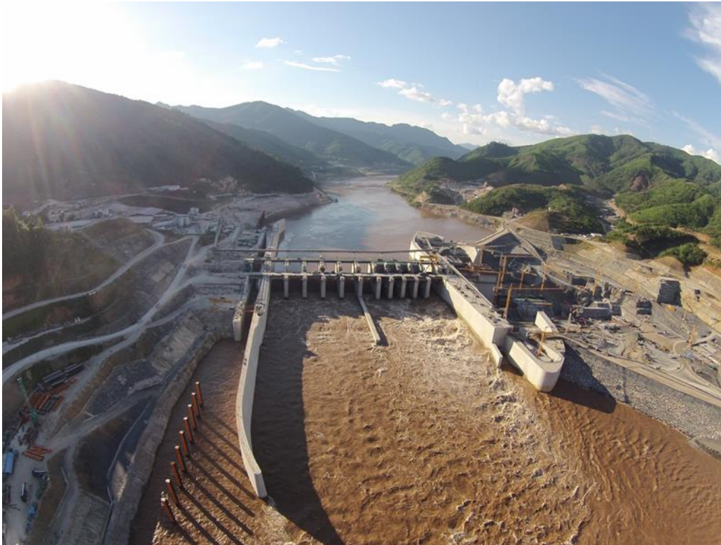
Figure 1: Xayaburi Hydroelectric Project - June 2015 (courtesy of Poyry Engineering Ltd).
