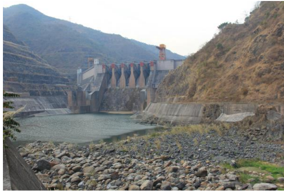
Photo 2-3 Dachaoshan Hydropower Project (Source www.flickr.com )
